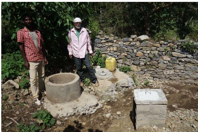
Biogas at Guhmi village - animal waste collector and latrine combine to provide gas for lighting and cooking. A 'by-product' of the sanitation and hygiene program!
